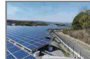
Solar Power System For High Speed Way
