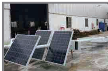
Solar Street Light System SAKO Engineer Commissioning
